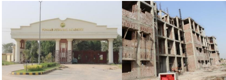
Under construction building of PJA at Kala Shah Kaku
