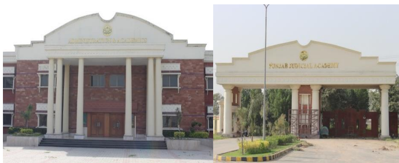
PJA new under construction building at Kala Shah Kaku
