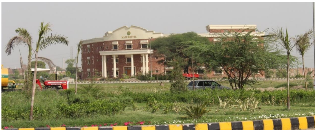
A view of new PJA constructed building at Kala Shah Kaku
