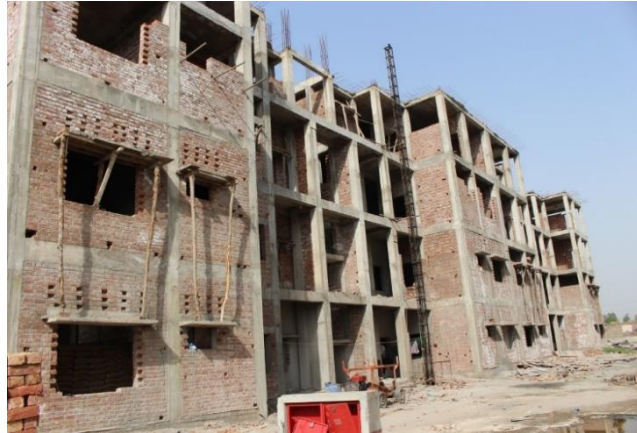
A view of new PJA under construction building at Kala Shah Kaku
